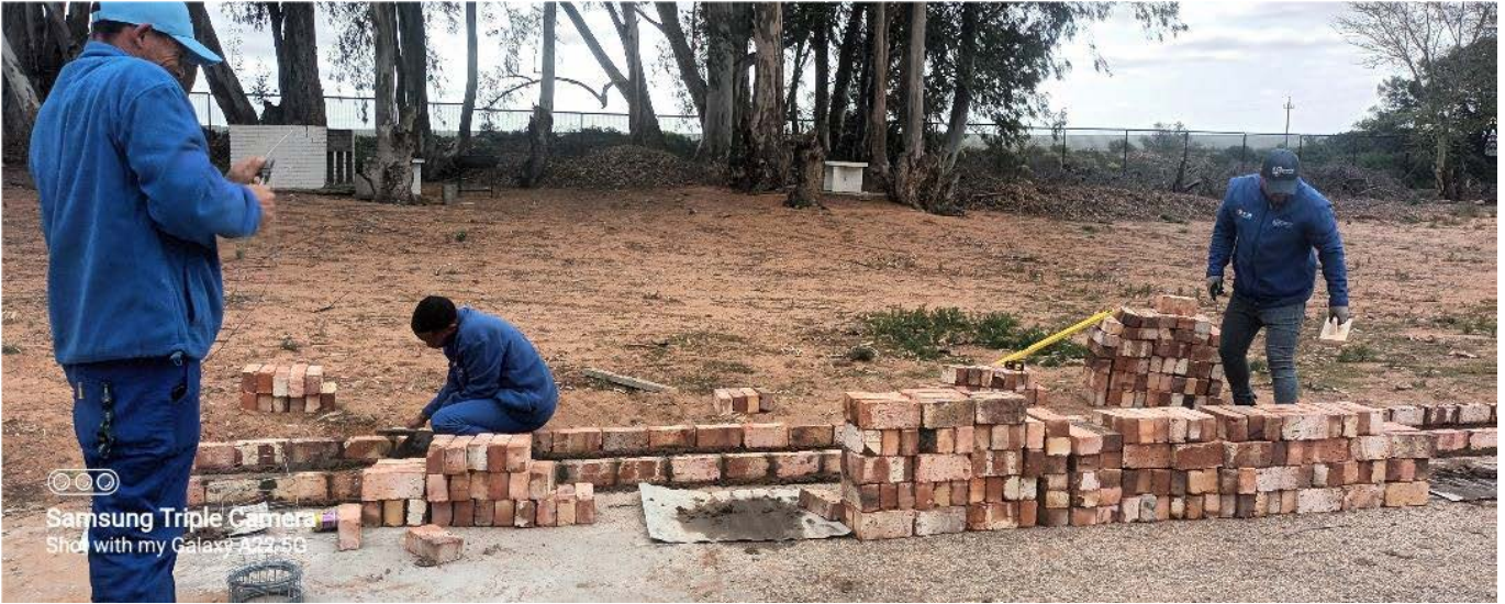
The EPWP Team building plant holder at the Koekenaap cultural facility
