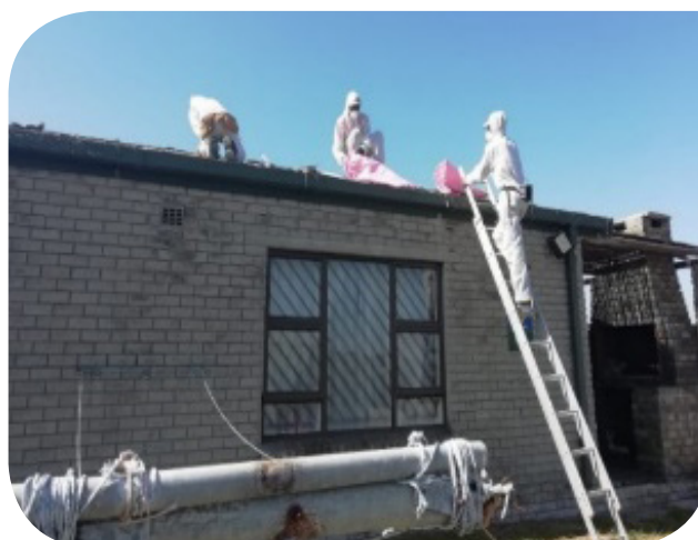
Experts in the handling of asbestos at the Melkbos cultural centre - fixing the roof of state-owned house
